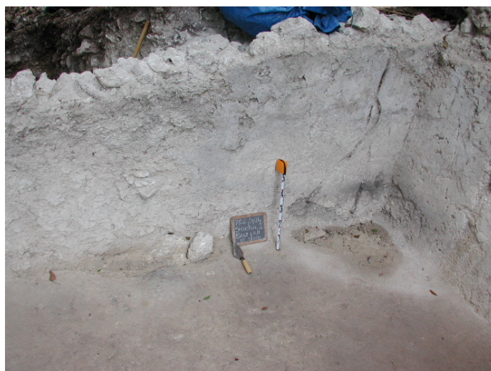
Figure 3.10: Structure 1, interior juncture of north and east walls.
