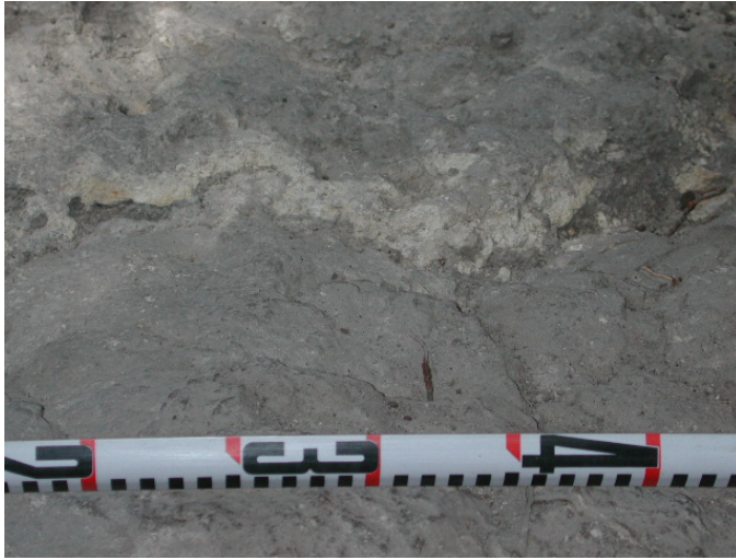
Figure 5.12: Close view of plaster lining over bedrock.
